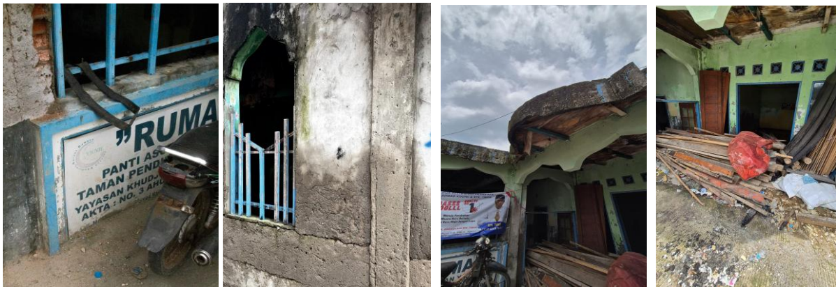
Figure 3. Current Condition of the Orphanage (2025, Captured by author)
