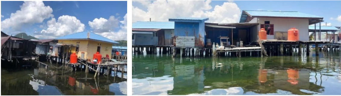
Figure 4. Condition of sanitation and clean water facilities in Tobati Village, 2024.
