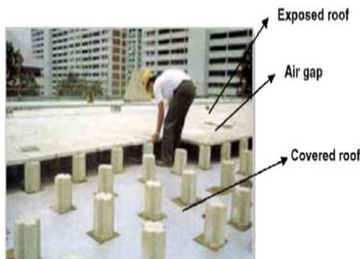
Fig.7 Secondary roof system construction, source: Wong & Li (2007)
