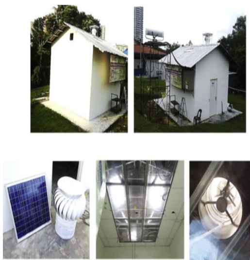
Fig.4 Innovative Roof Structure, source: Al-Obaidi, Ismail & Abdul Rahman (2013)
