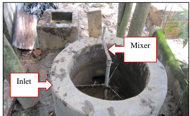
Figure 7 The complete structure of the digester and hydraulic chamber
