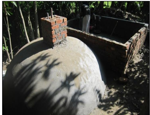
Figure 7 The complete structure of the digester and hydraulic chamber
