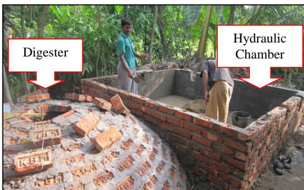
Figure 6 The construction of outer structure of the digester and hydraulic chamber
