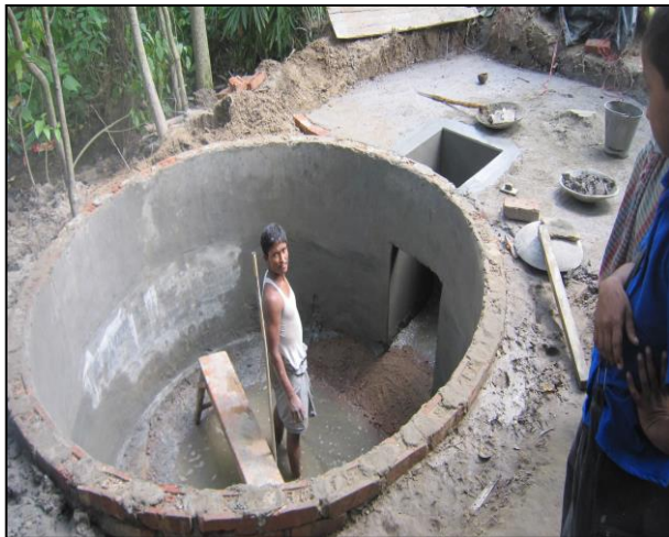
Figure 5 The base construction of the digester and hydraulic chamber
